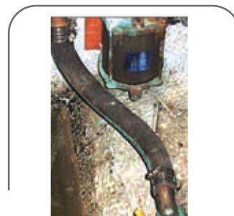
Clamps installed with screw tightening heads in line. It is recommended to offset as see below.
